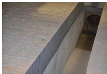
Prepared Filter Floor After Demolition
