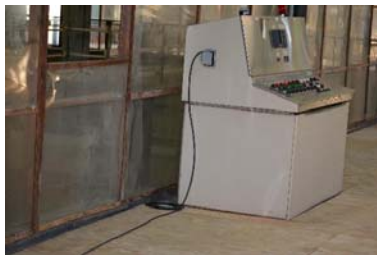
1930 Filter Gallery Old Partitions
