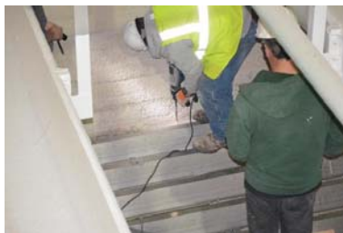
Installing New Underdrain System
