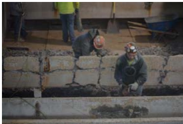
Demolition of Wash Water Troughs
