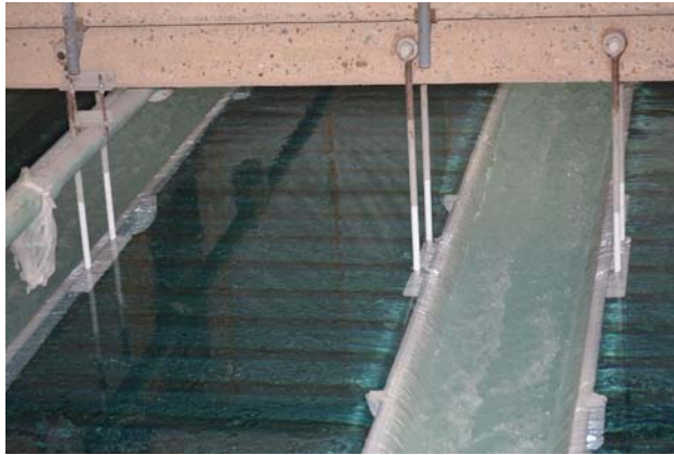
Hydraulic Distribution Testing on New Underdrain System
