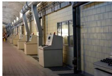
New Partitions and Ductwork in 1930 Filter Building
