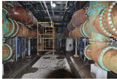
Existing 1958 Filter Pipe Gallery
